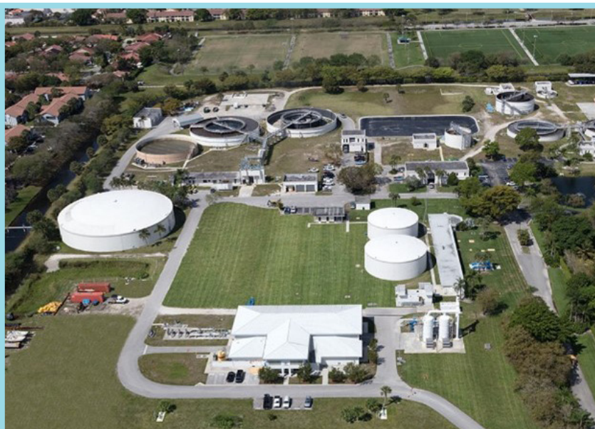
Plant Site with Water Plant in Foreground with LS facilities removed and Wastewater Plant in Background.
