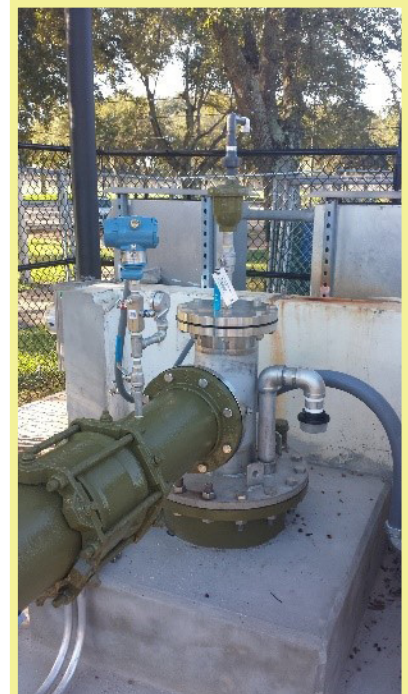
Modified Well 6 Wellhead
