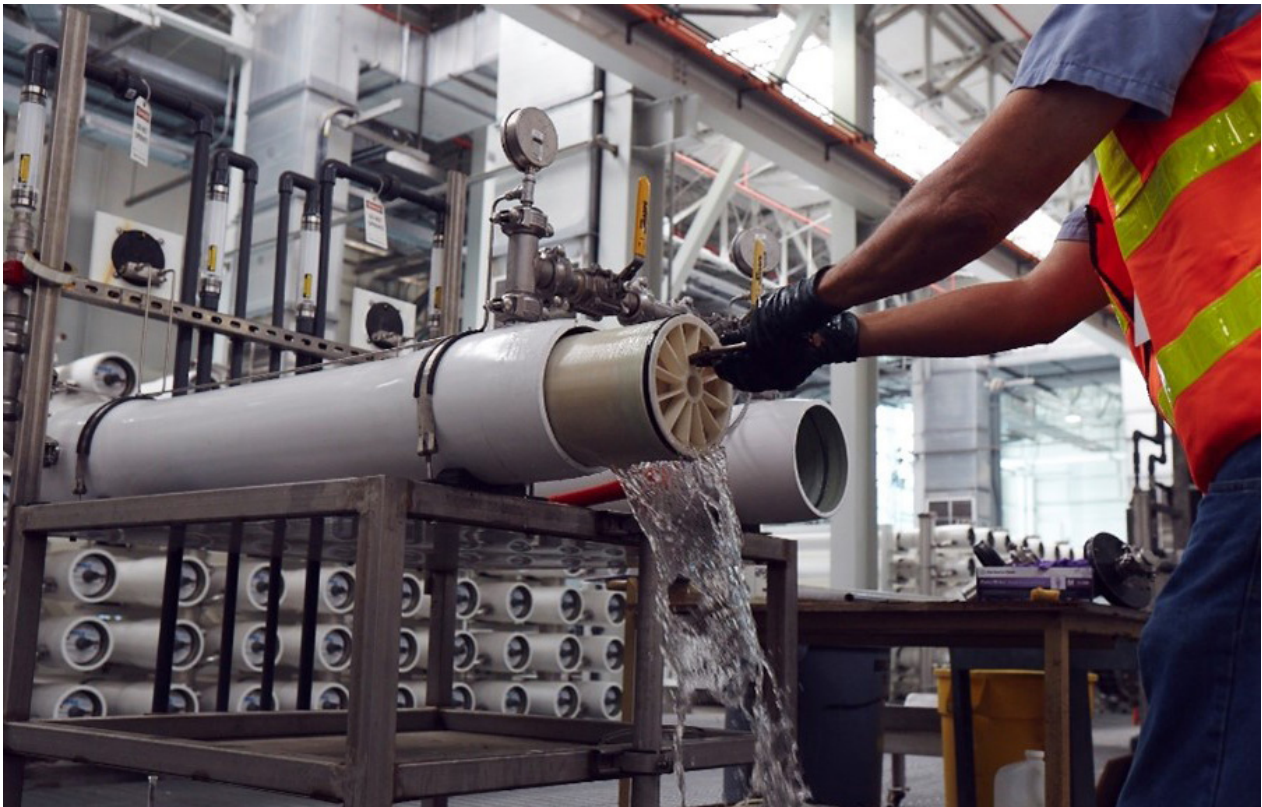
Image 4: FILMTEC™ RO membrane being changed at OCWD facility
