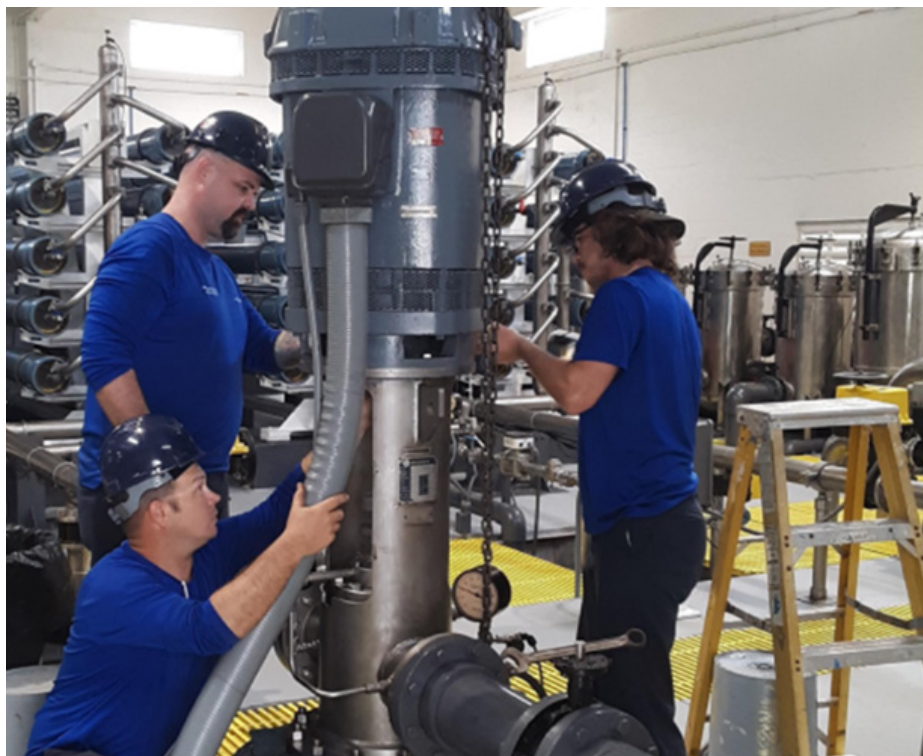
IWA plant operators work together to align a pump at the RO membrane plant.
