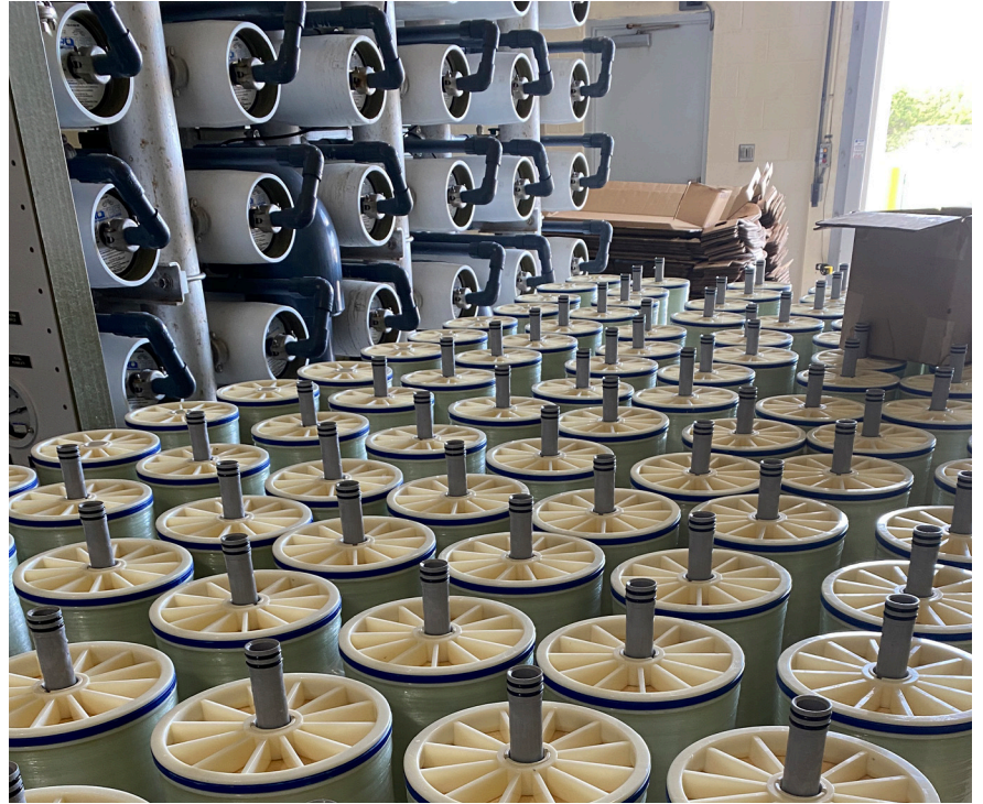
Unpacking of New Membrane Elements for Installation
